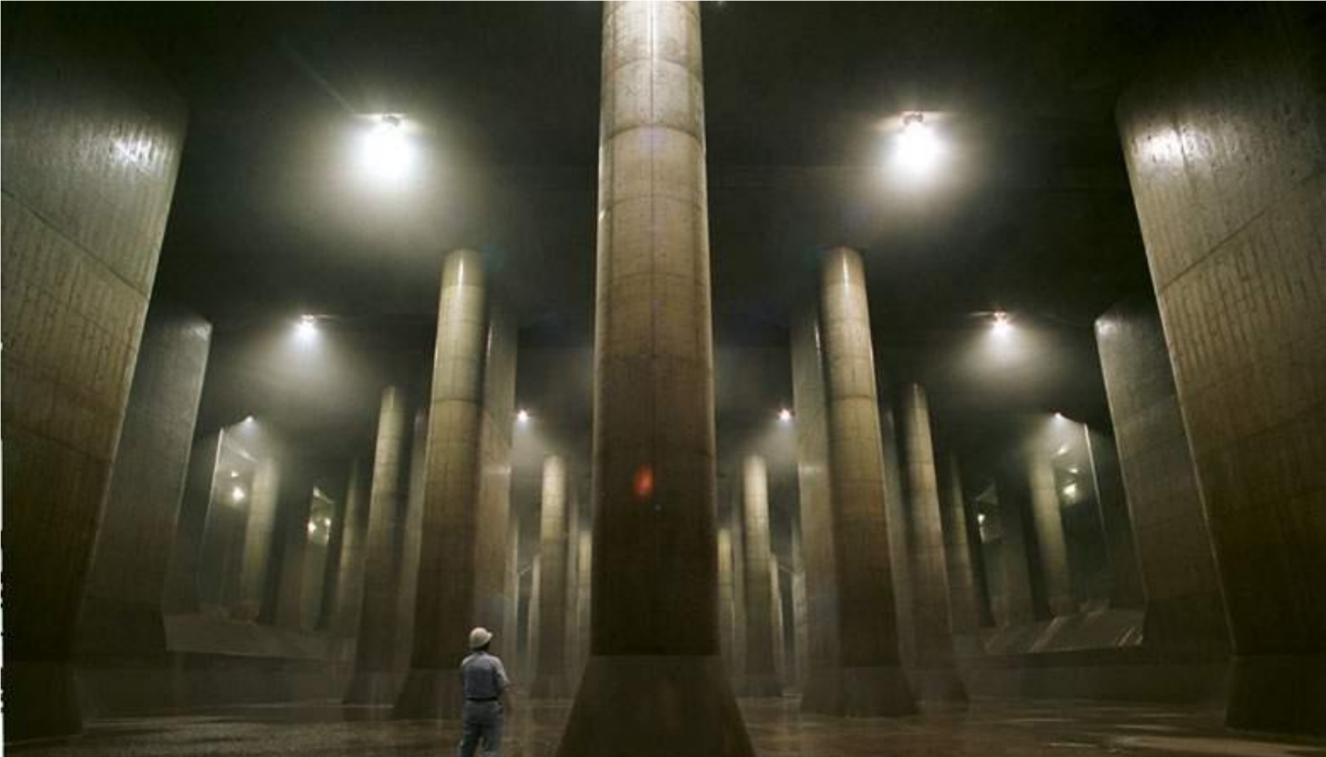
Tokyo: Underground stormwater retention reservoir
